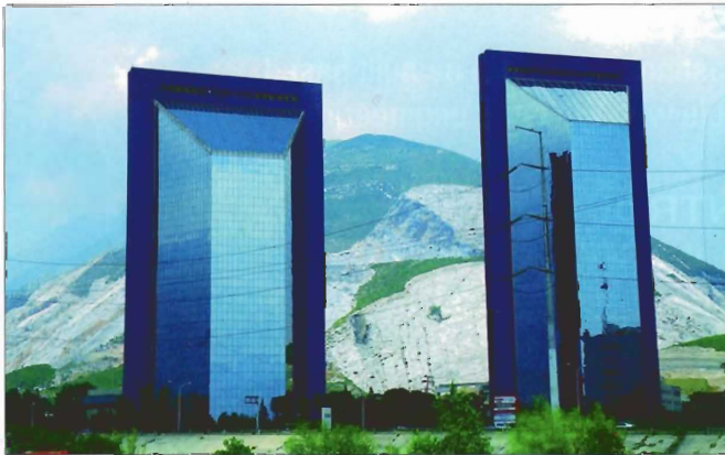
Figure 2. Cuprum used 6063-T5 clear anodized aluminum for the curtain wall in the "Oficinas en el Parque" towers in Monterrey, Mexico.
